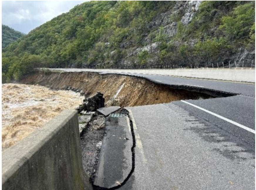
Figure 1 A ground level image of the damage of Interstate-40 at Pigeon River Gorge caused by Hurricane Helene and rising river waters.
